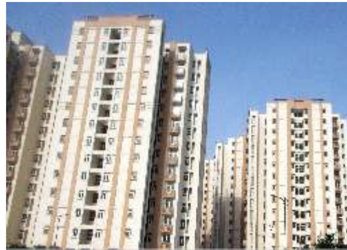
SHREE VARDHMAN mantra GOLF COURSE EXTN. ROAD SEC-67, GURGAON 11.26 Acres Group Housing Sector-67, Gurugram
